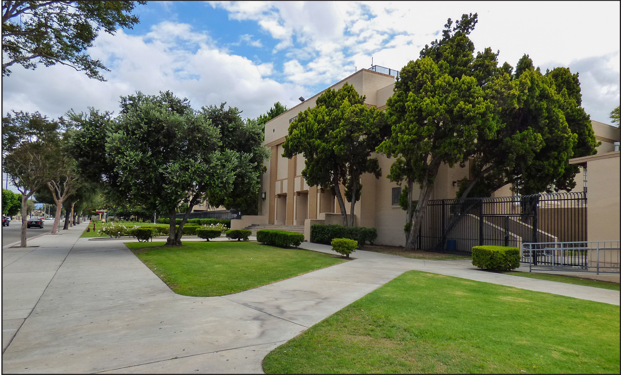
Photo 3. View looking northeast toward Westover Hall (Auditorium), (Building 2) from sidewalk on Miles Avenue.
