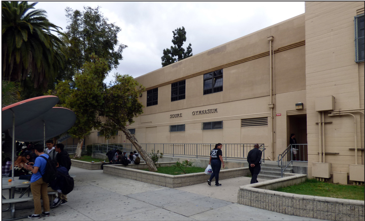
Photo 7. View looking north toward Gymnasium (Building 13) from Belgrave Palm Court.
