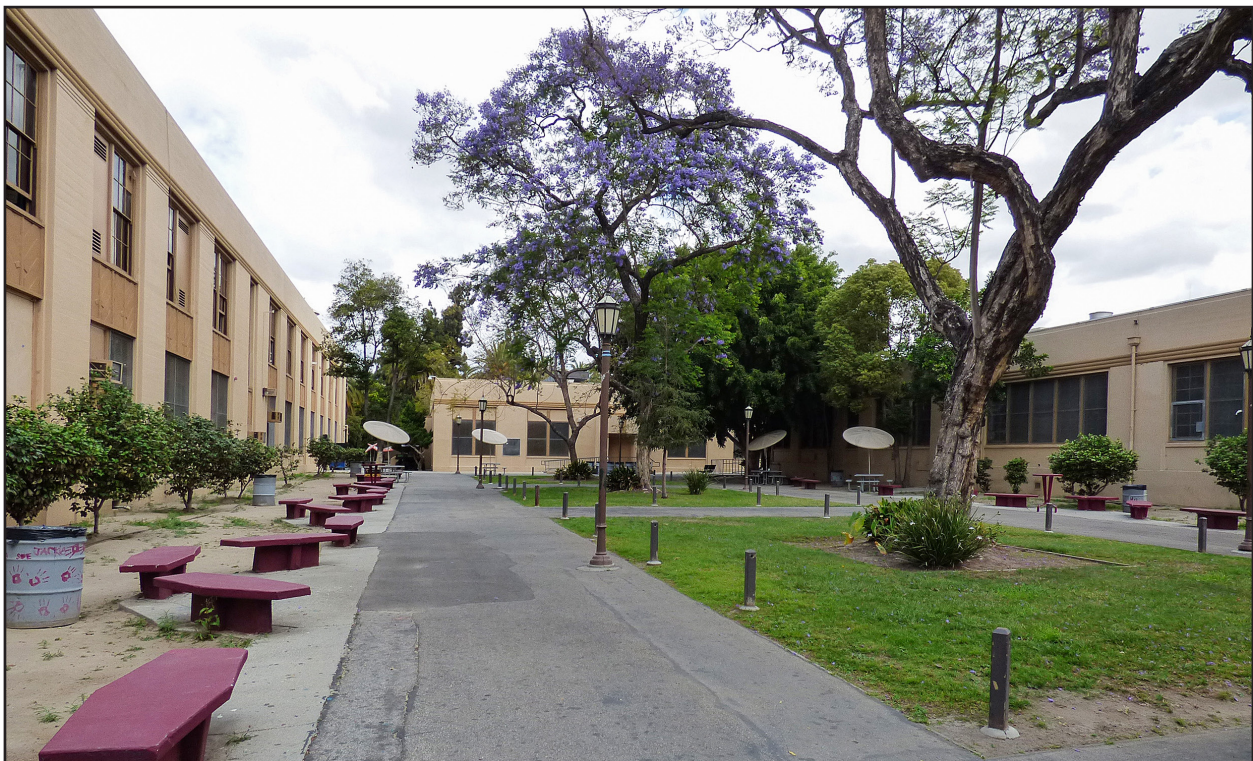
Photo 6. View looking northeast toward Stockton Court from corner of Administration (Building 1) shown on left. Cafeteria (Building 3) is in background center and Home Economics (Building 4) is on the right.
