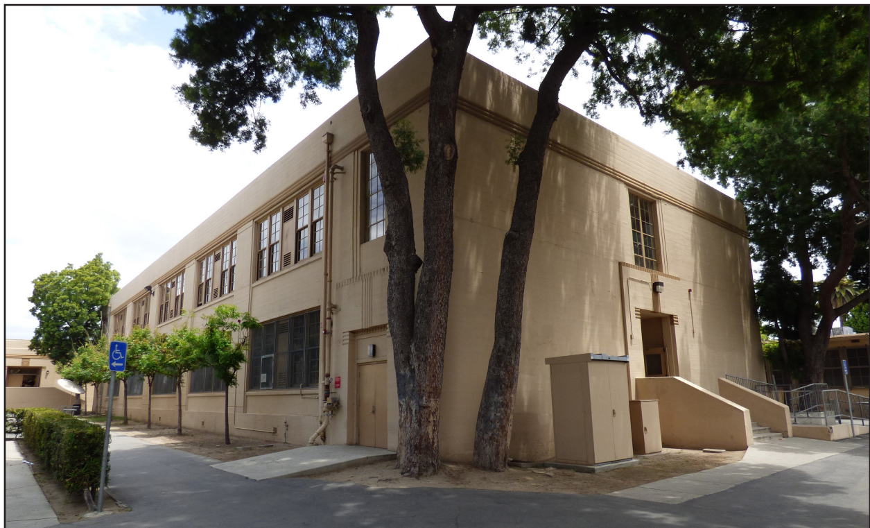
Photo 2. View looking northeast toward Annex (Building 8) from Music (Building 18).
